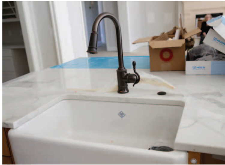
Hot water is never more than a few seconds away, thanks to the loop supply system. Less water is wasted waiting for hot water.
