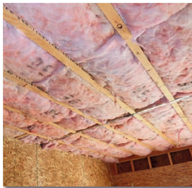
Figure 3: Insulated floor over garage
