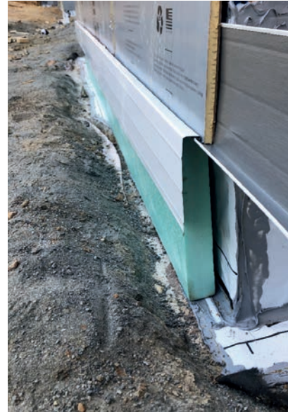
Figure 5: Slab Edge insulation with flashing and protection.
