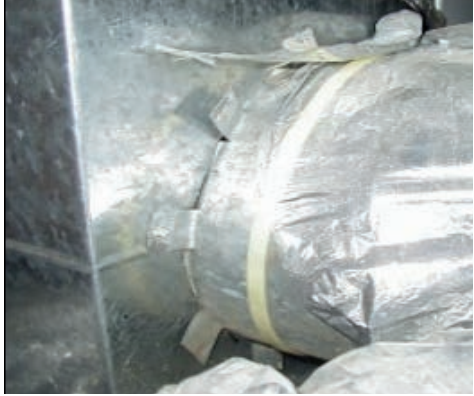
Figure 5: Unsealed tabular duct takeoff
