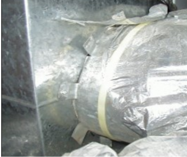
Figure 5: Unsealed tabular duct takeoff
