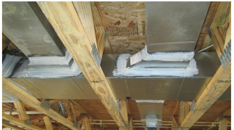
Figure 4: Well sealed supply-to-trunk connection
