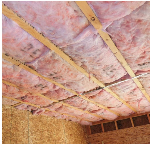
Figure 3: Insulated floor over garage
