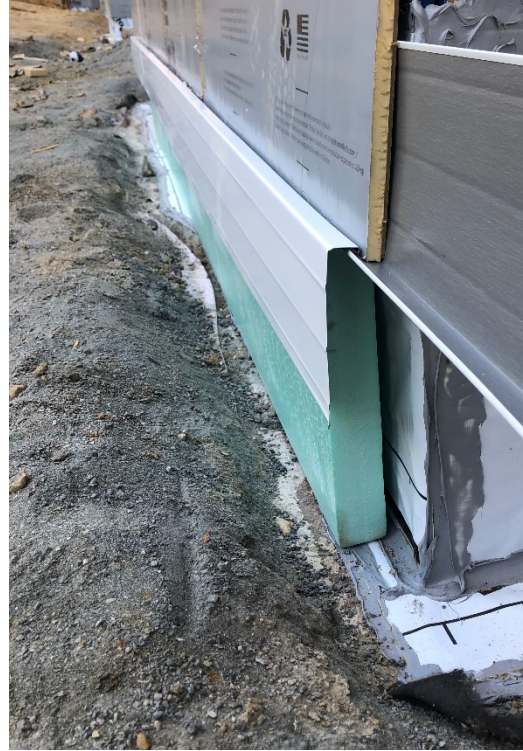
Figure 5: Slab Edge insulation with flashing and protection.
