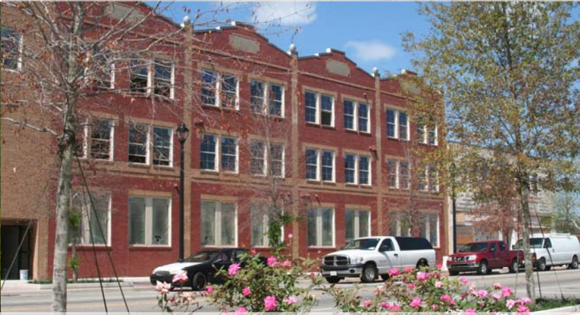
NNRHA - Jefferson Brookville Rehab
