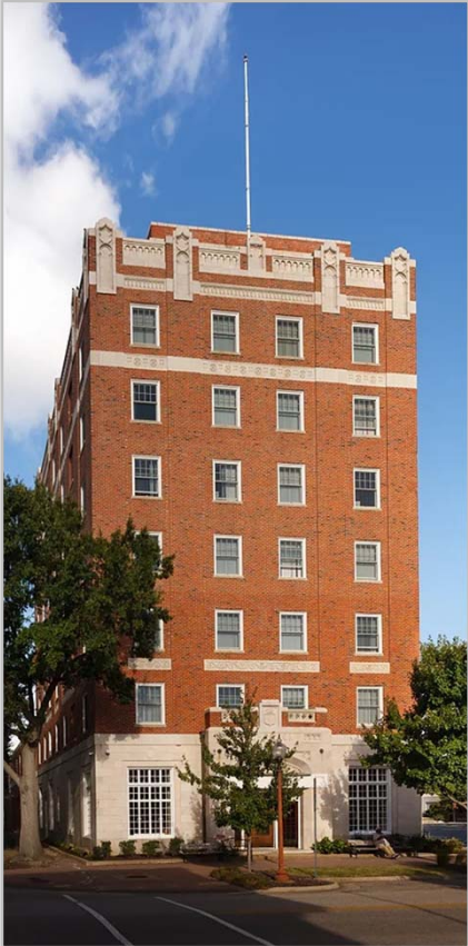
Warwick SRO Newport News, Virginia Photo credit: Community Housing Partners
