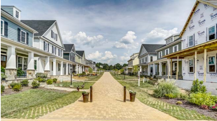
Stony Point Design/Build - Riverside Village
