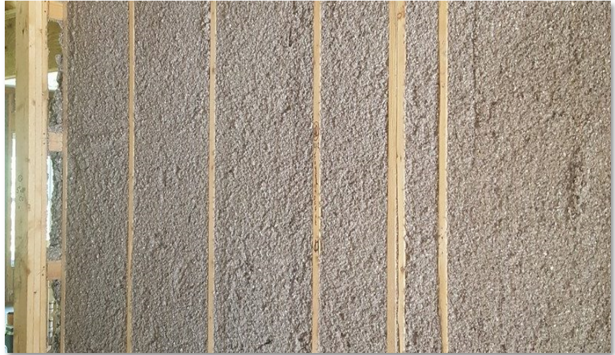
Figure 3: Damp-spray cellulose insulation in wall
