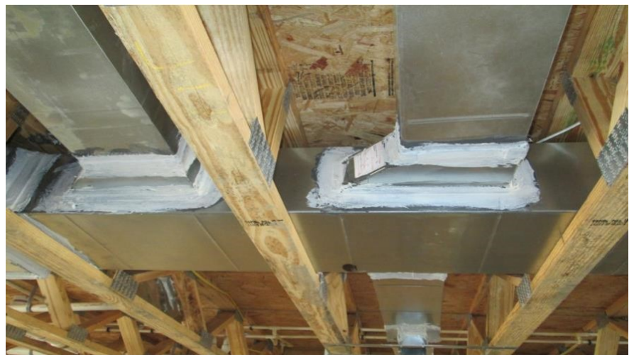
Figure 4: Well sealed supply-to-trunk connection
