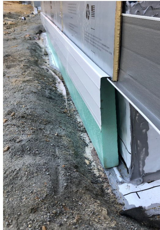
Figure 5: Slab Edge insulation with flashing and protection.
