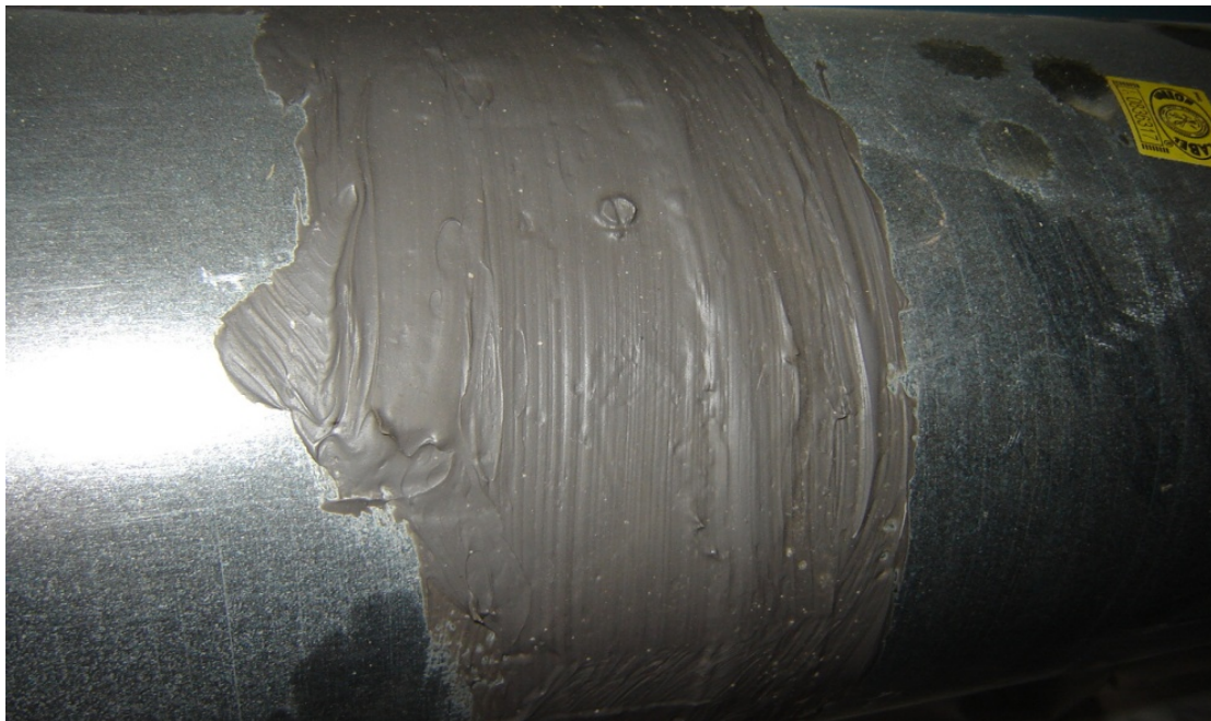
Figure 7: Mastic paste used as permanent seal – “thick as a nickel”
