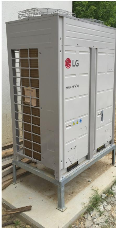
Figure 4: VRF outdoor unit is set on a pad on the perimeter of the building.
