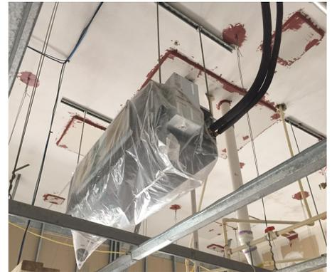
Figure 2: Diligent ceiling unit airsealing by KBS improved the compartmentalization and overall airtightness of each apartment, reducing energy consumption, and improving indoor environmental quality.
