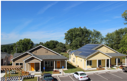
East elevation of Grissom Lane Apartments. Photo Credit: Community Housing Partners
