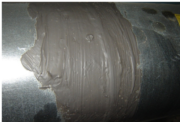
Figure 7: Mastic paste used as permanent seal – “thick as a nickel”
