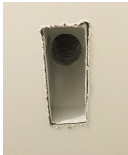
Figure 2: Increased duct and envelope leakage if left unsealed
