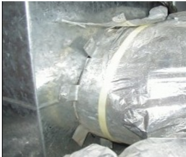
Figure 5: Unsealed tabular duct takeoff
