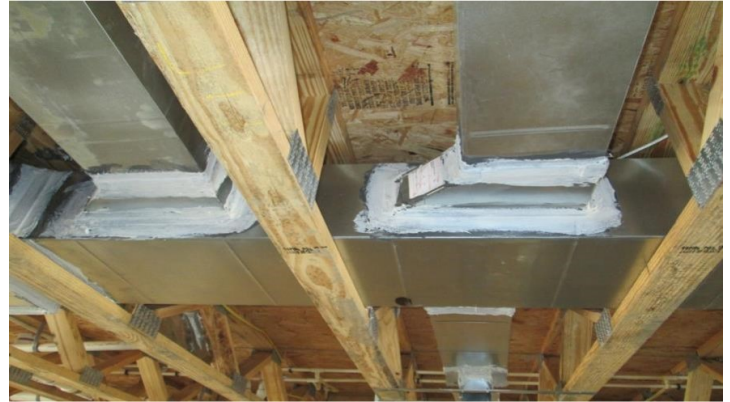
Figure 4: Well sealed supply-to-trunk connection
