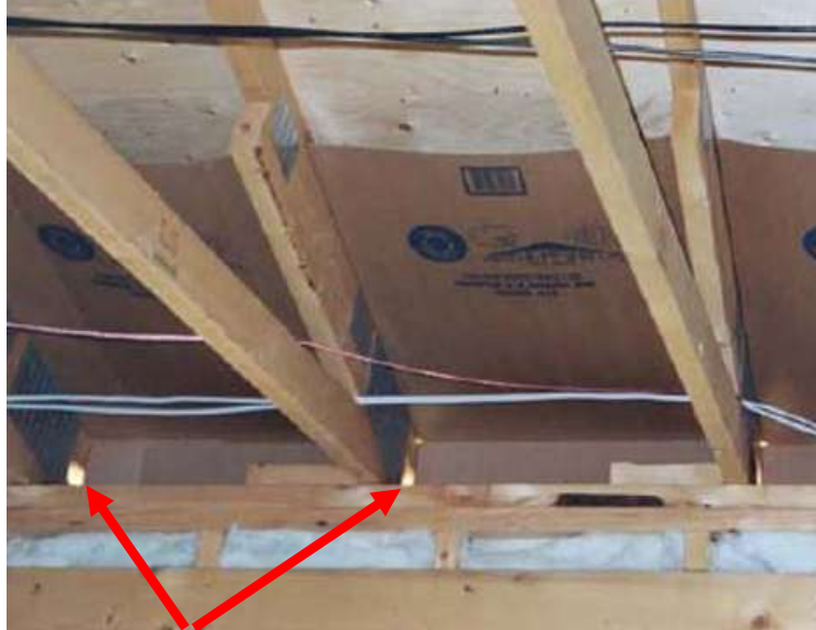
Image: daylight shows gaps to be caulked around cardboard baffles to eliminate air intrusion; photo: Viridiant
