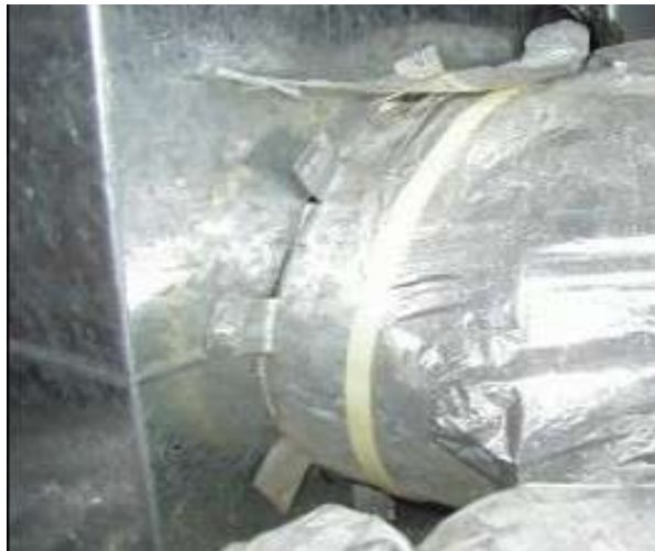
Figure 5: Unsealed tabular duct takeoff
