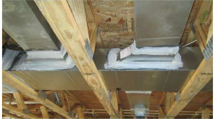
Figure 4: Well sealed supply-to-trunk connection
